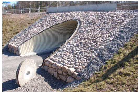
Foto 4. Betoonalusel munakividega kindlustamine (foto: Sten-Eric Lager [29])
